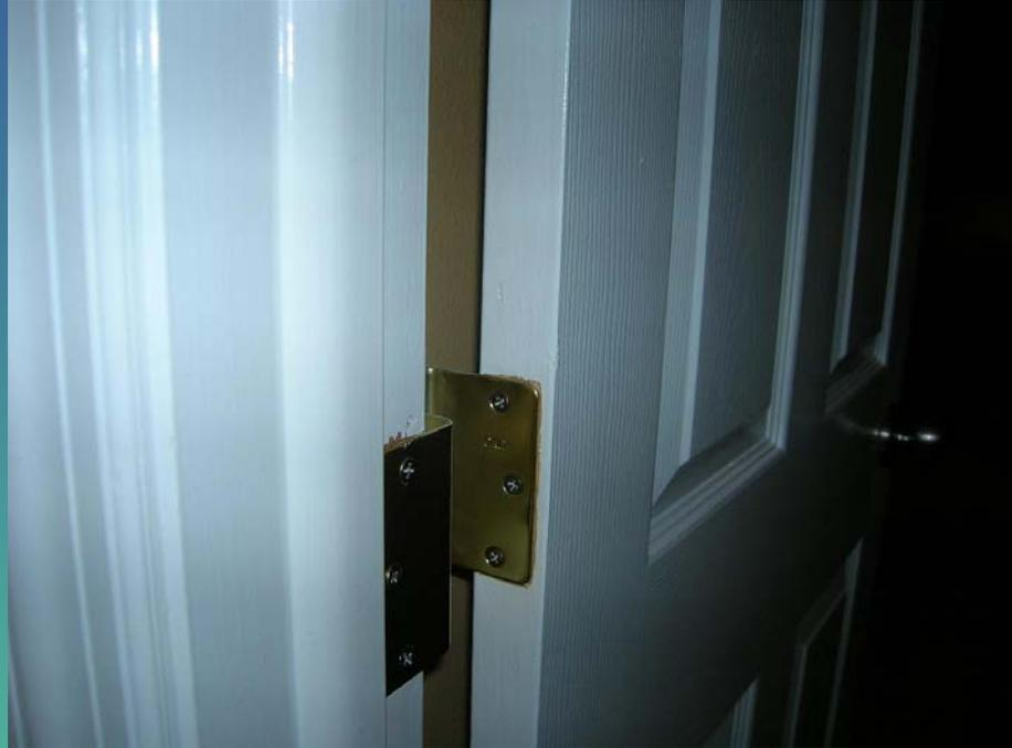
Widening doors is very expensive, I found these “Swing away” hinges on e-bay. You install them in place of the standard door hinge and it allows the entire door to swing away giving you extra width at the door way.
